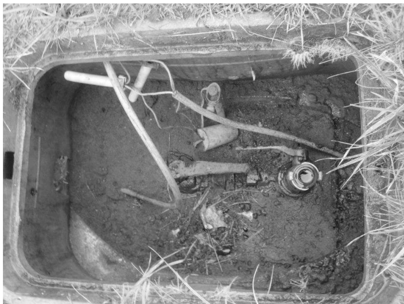
Green isolation valves Note; condition of handles and access to components (assemblies are certainly showing their 24+ years)
