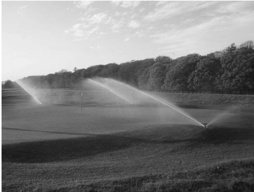
Green sprinklers in operation – note poor spacing and reduced pressure
