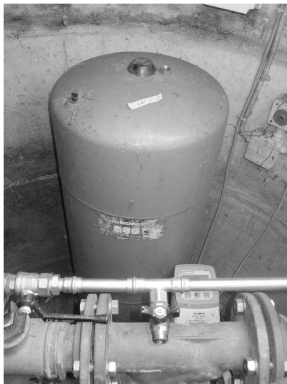
Pressure vessel in well head chamber [old]
