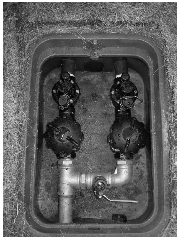
Typical Tee solenoid valve assembly – 2018 [example photo]
