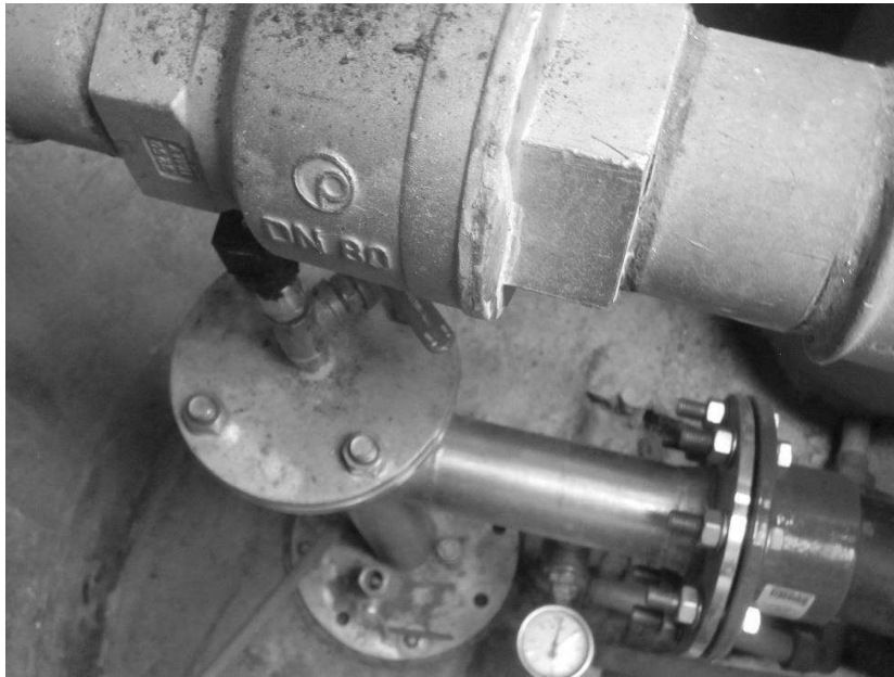
Irrigation borehole well head manifold [new]
