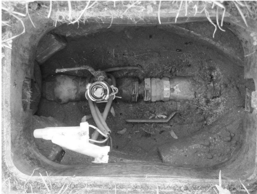
Green isolation valves Note; condition of handles and access to components (assemblies are certainly showing their 24+ years)
