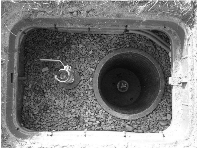
Typical Green isolation valve assembly – 2018 [example photo]
